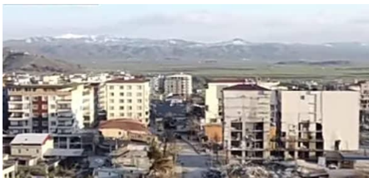
Fig 14. Nurdagi after February Earthquake 2023, Aljazeera news
